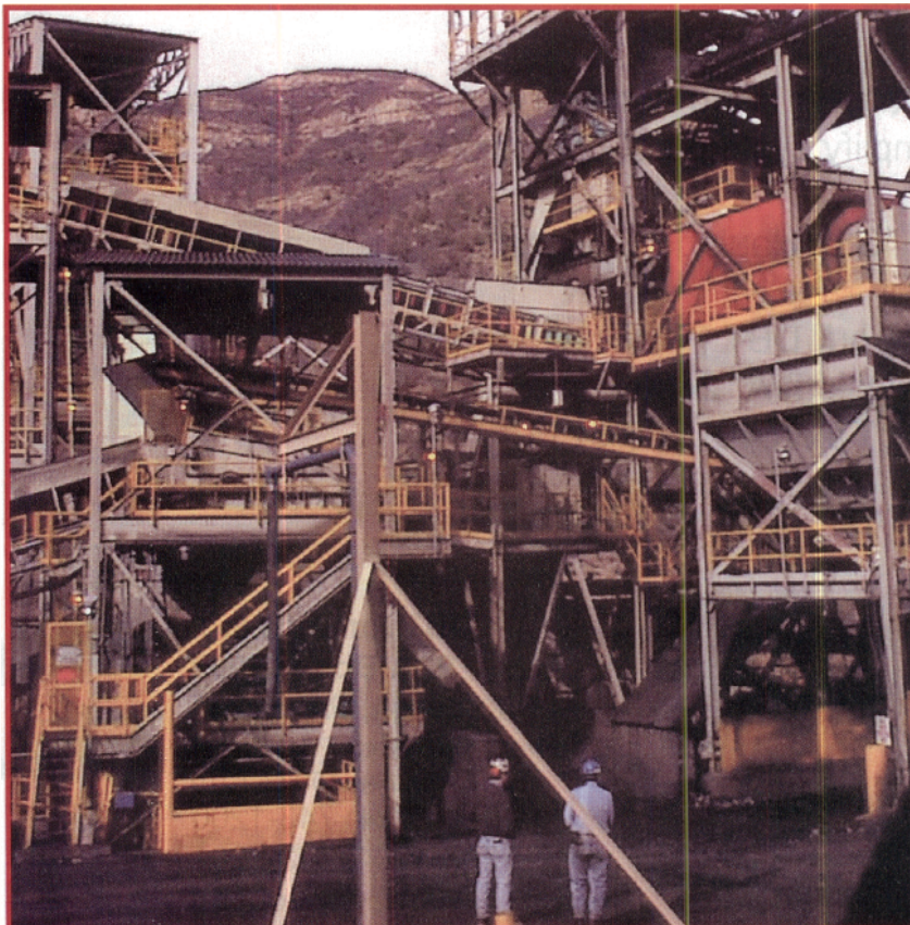
To solve transfer plugging problems, West Elk employed a computer simulator that used discrete element modeling.
